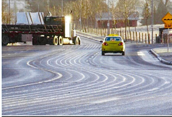
Figure 5.1.8 - Application of deicing agents on road ( www.harmonydeicing.com )
