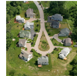
Bioretention area in Waterford, CT (middle)
