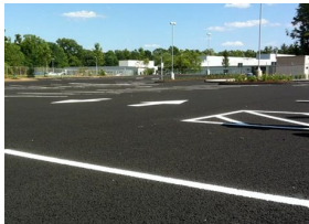
Pervious asphalt at Goodwin College
